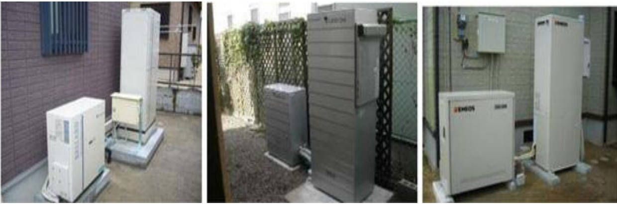
Figure 2- 9: Pictures of installation site.
