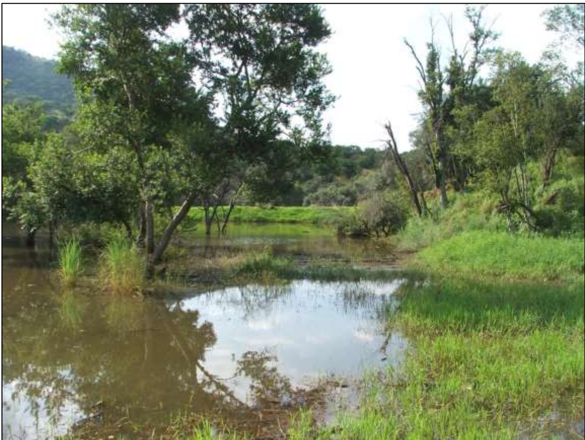
Figure 7.28. View of Vocifer Dam on Mogale's Gate Biodiversity Centre.
