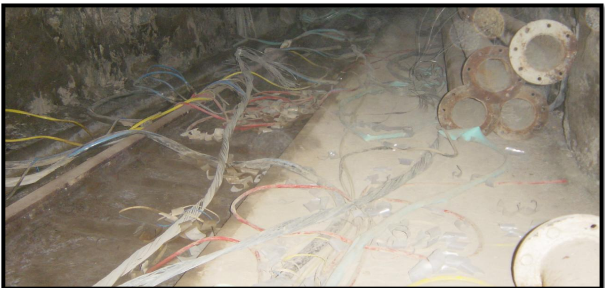
Figure 3.3: Photograph of redundant underground mining operation after copper cable theft
