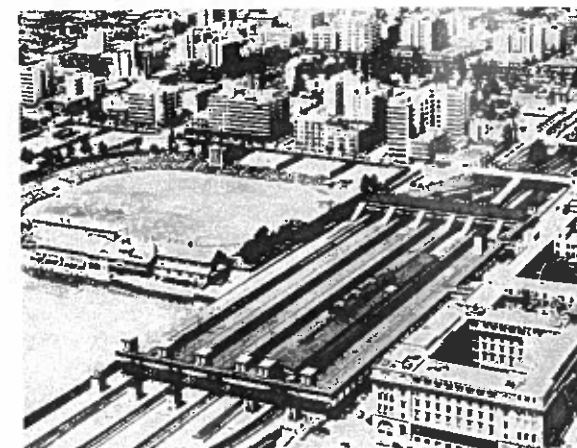
Top right: A sketch plan illustrating the location of the railway museum in Newtown — adjacent to the northern railway lines. The possible adjustment of the proposed Yale Road extension and modifications to the routes of Wolhuter and Carr Streets are shown. By courtesy of Gallagher Aspoas Poplak Senior, urban designers Right: The sequence of photographs illustrates the station building in a changing urban context — in the 1920s, additional lines are being constructed; in the 1930s, the south station building, designed by Leith & Moerdyk, is complete; and in the 1940s the SAR regional offices (in the foreground) are complete
