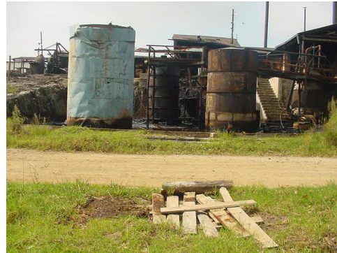
d) Sampling point at effluent trench
