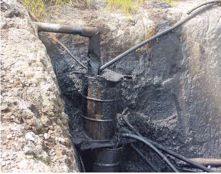
g) Effluent from trench and discharge point
