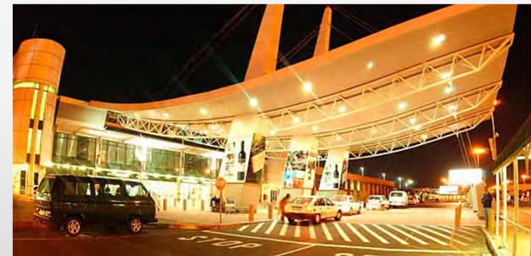
Cape Town International Airport (R1,6 billion)
