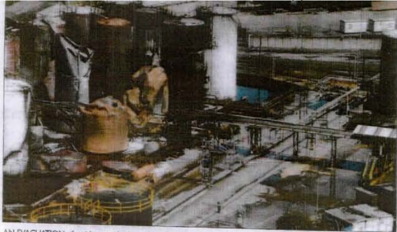
AN EVACUATION of residents took place after a fire broke out in some of the tanks at Island View Storage
