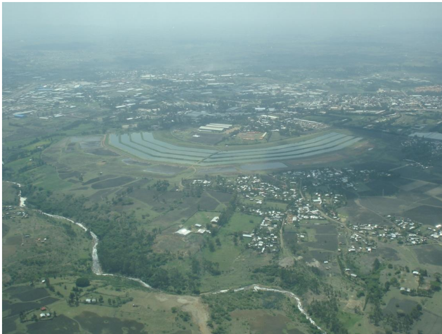
Fig. 5.6 The treatment plant in the vicinity of the Akaki aquifer
