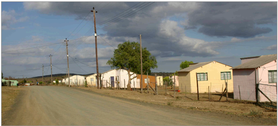
Figure 69 Photographs of typical houses and street scene in Glenmore village.
