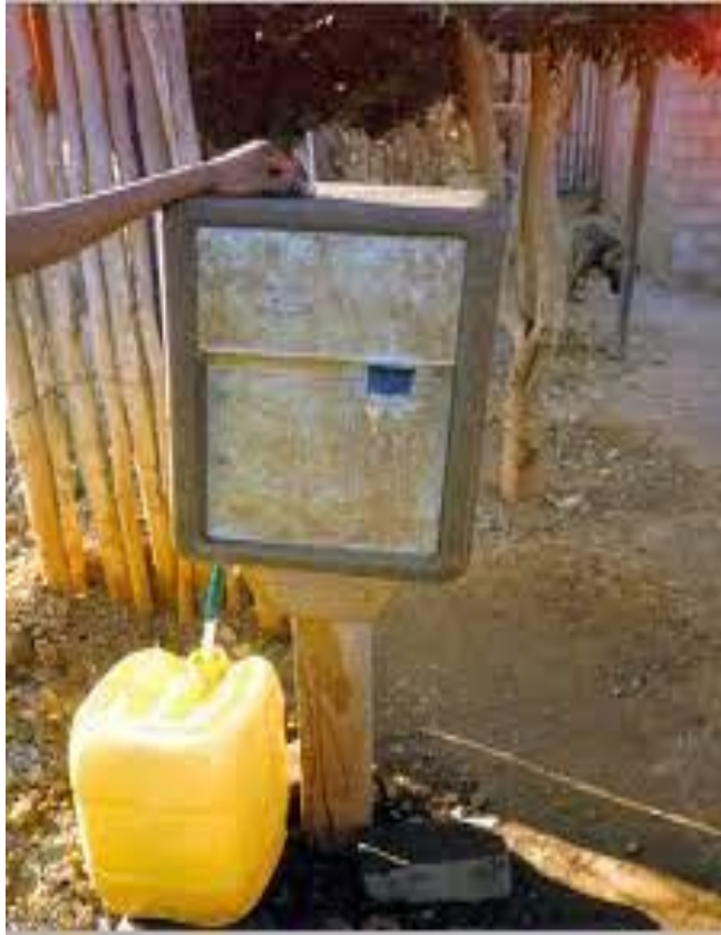
Figure 4.3: Prepaid Water System (Karuaihe & Wandschneider, 2018)
