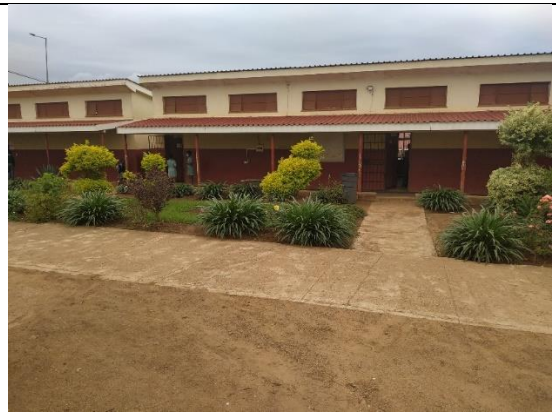
Photo 10: Adequate basic buildings at school P1
