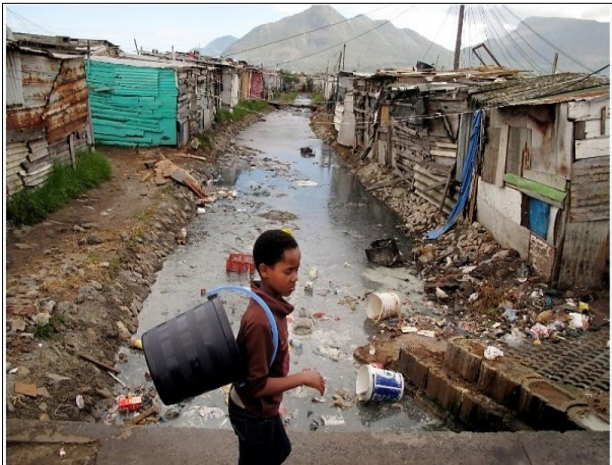
Figure 4. 2: Masiphumelele Sewage Canals
