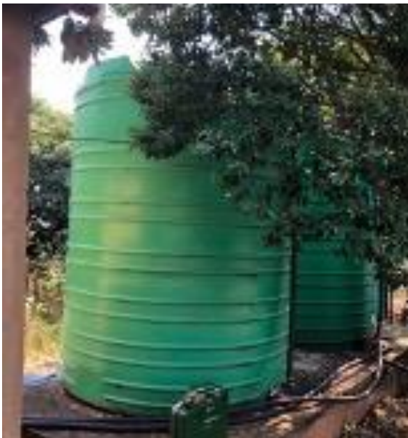
Water storage tanks – water comes from reservoir into tanks to be pumped for irrigation or gravity fed if topography of land facilitated it (Business 6, 9).
