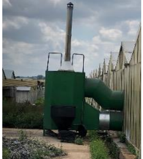
Photo 40 – 41 – Boilers used for heating greenhouses in winter
