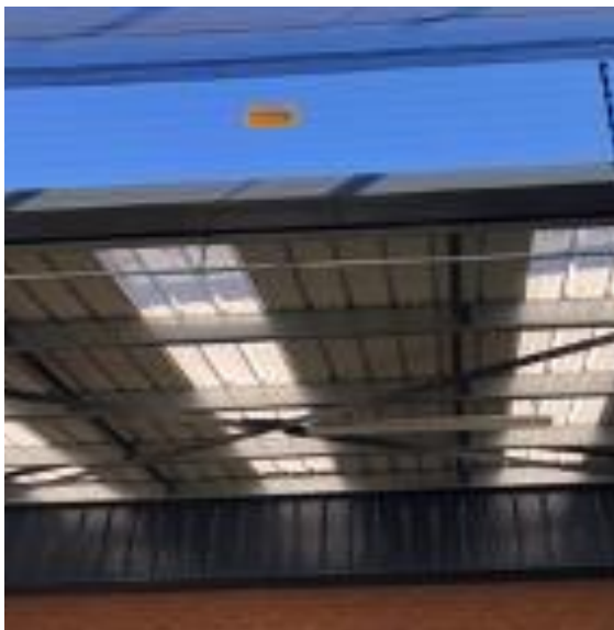
Use of natural lighting by changing roofing materials (Business 2, 17, 34, 19,
