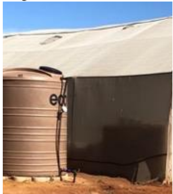
Water storage tanks – water comes from reservoir into tanks to be pumped for irrigation or gravity fed if topography of land facilitated it (Business 6, 9).
