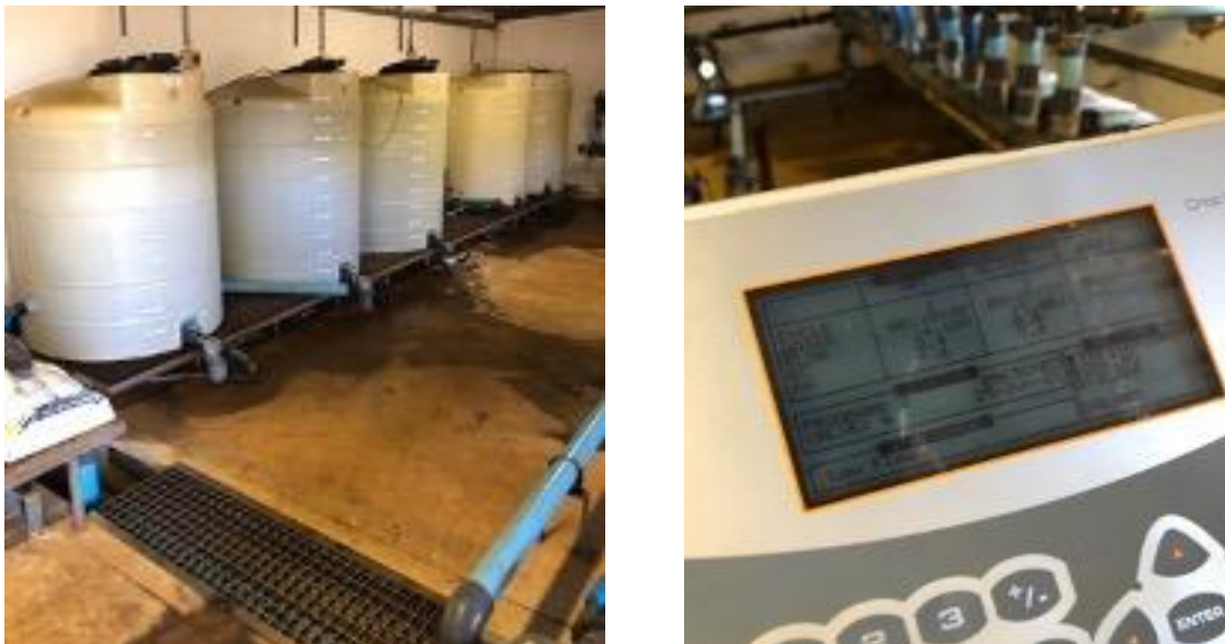
Photo 15 - 16 – Using technology to monitor fertiliser levels in tanks and irrigation
