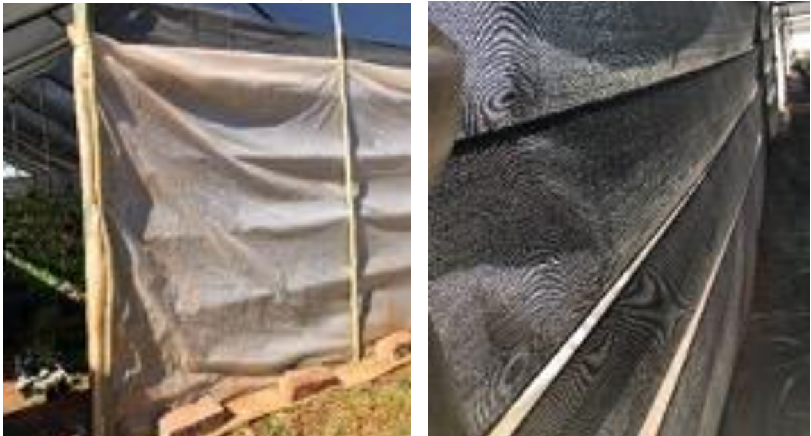
Photo 29 – 31 – Fabric or plastic screens around sheds for protection
