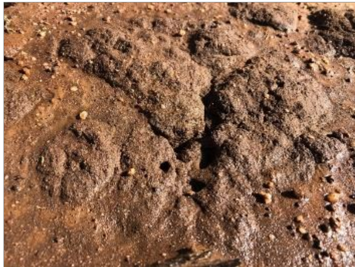
Figure 5.13: Cracks between dry strong Prismaeutanic structural units exposed after starting to wet the soil
