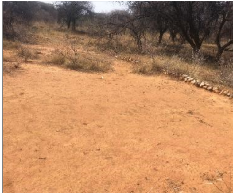
Figure 3.9: Gabion-like structures installed along contours at the degraded areas
