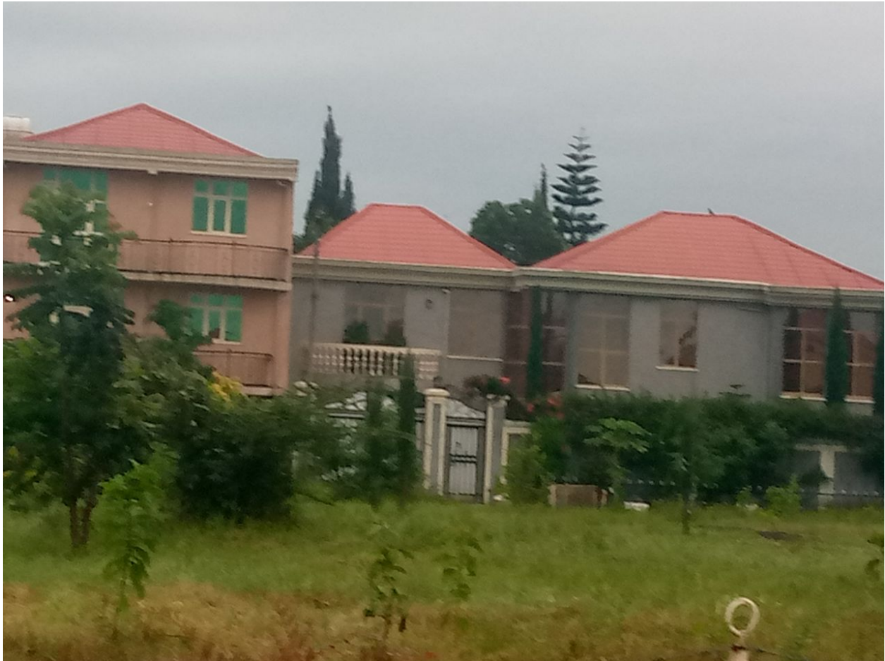
Figure 5.2 Current urban residential buildings in Bishoftu city (Source: own camera)
