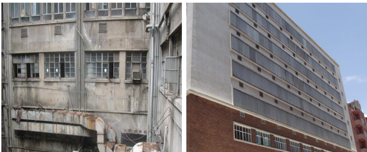
Figure 1: Before and After refurbishment – AA House
