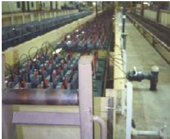
Fig. 6.9 Formation by soaking the batteries in water <math><30^\circ\text{C}</math>
