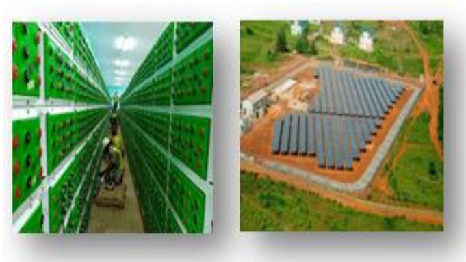
Fig 2.9 Telecommunication/Solar Integration of lead acid batteries.
