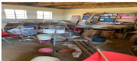
Picture E2: Classroom used as storage
