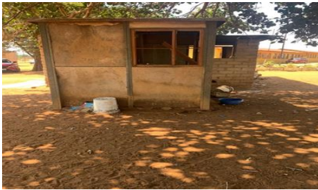
Picture Q3: Small house container
