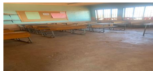
Picture V: Classroom
