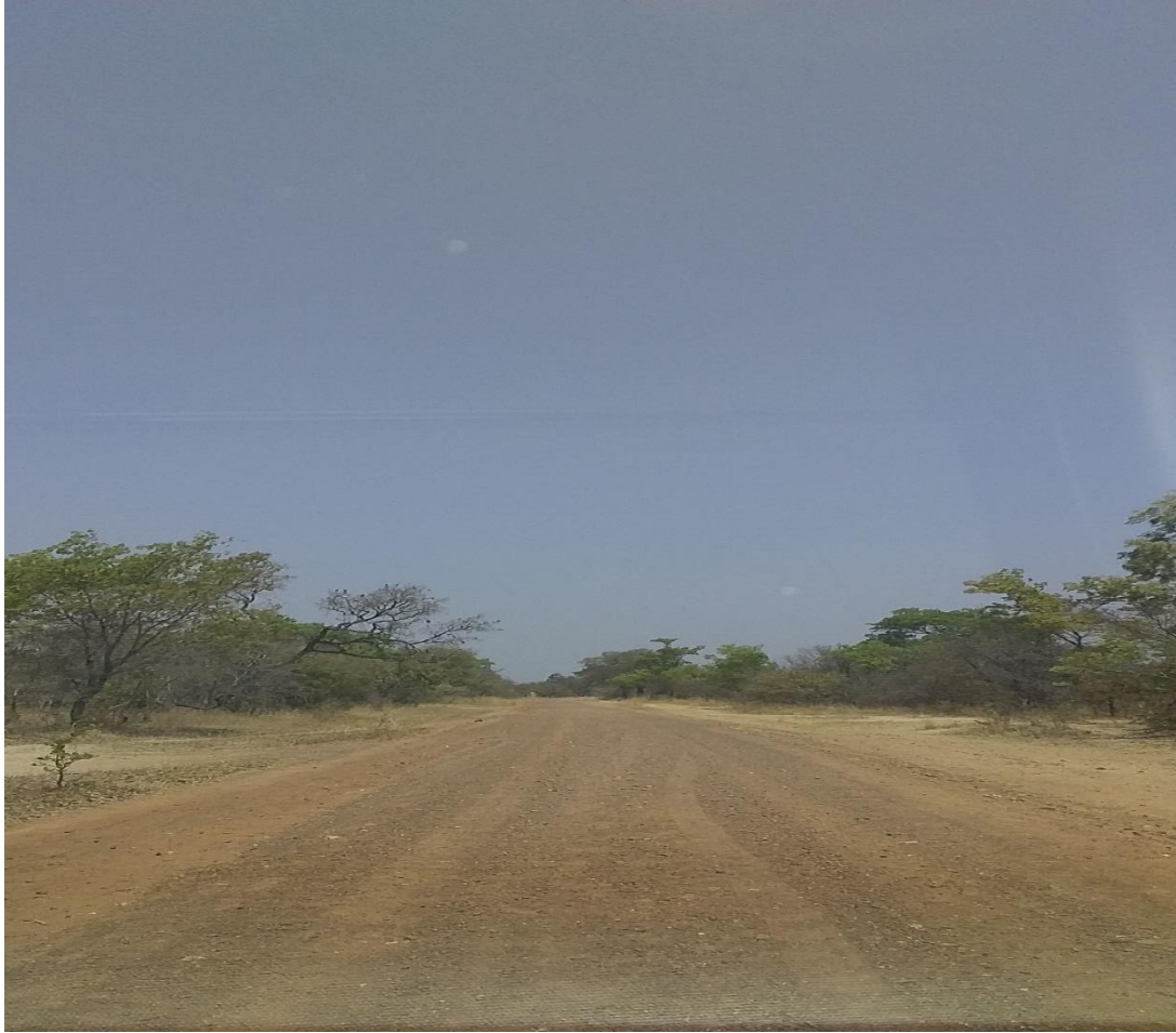
Figure 5.3: Pakame, Chachacha and Tongogara connection road that has been graded nicely.
