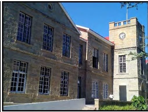
Figure 2.3: The main educational building at Lovedale 2018. 395
