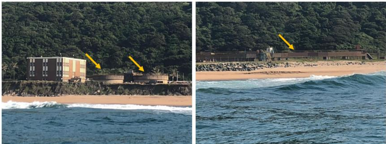
Plate 9. Pumping station for sewerage and industrial wastewater outfall pipelines in the South Durban basin.
