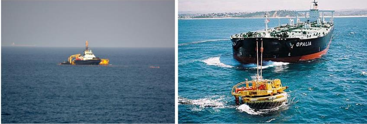
Plate 10. Single Buoy Mooring (SBM) located in the South Durban basin for pumping crude oil from super tankers to the inland petrochemical refineries.
