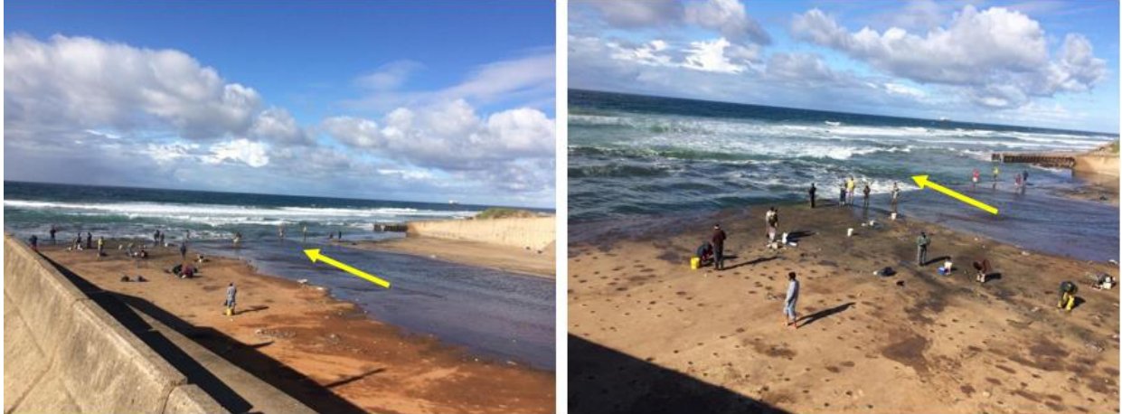
Plate 8. Storm water canals carrying discharges from South Durban industrial basin draining into the ocean that are popular for shore-based line fishing.
