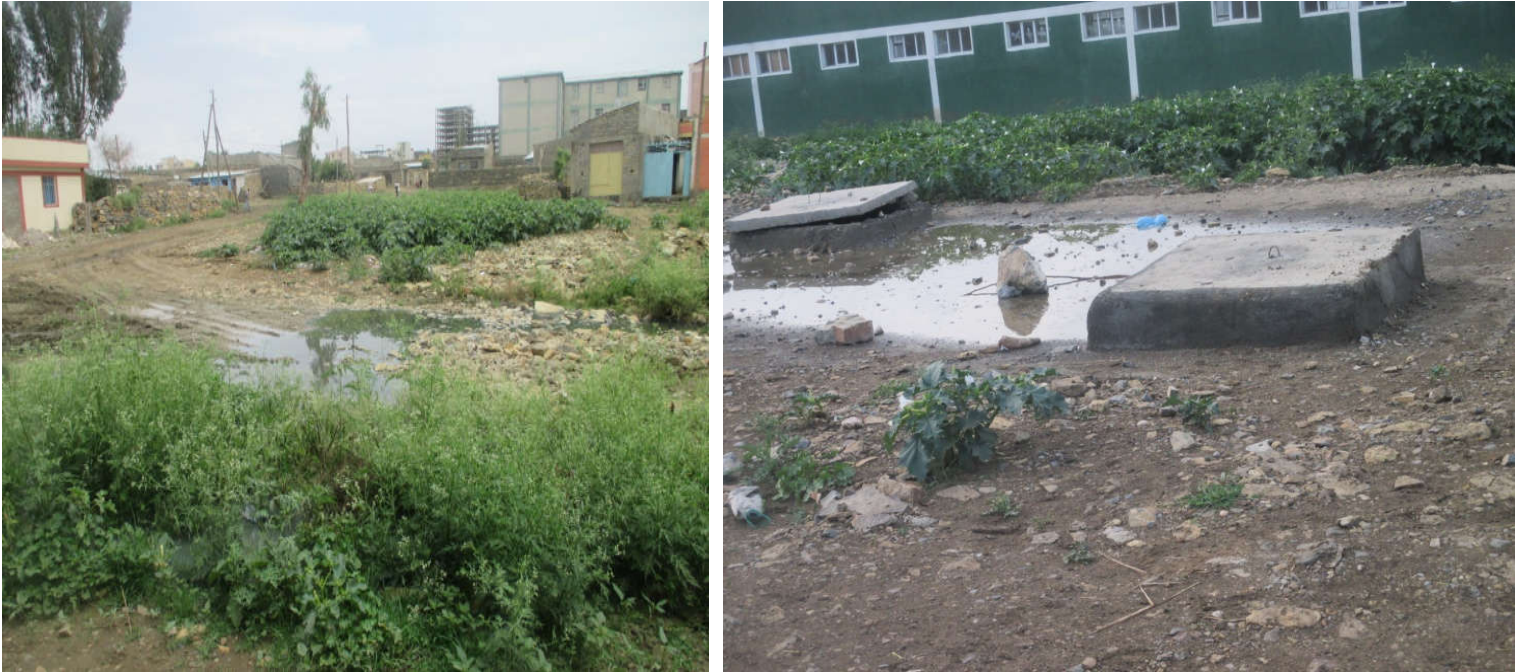
Figure 7: Spill over of septic tank in Kebeles 18, Mekelle City
