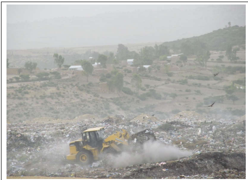
Figure 16: Loaders leveling the heaps of waste in the landfill of Mekelle City Sources: Photo captured during field observation, 2015/16
