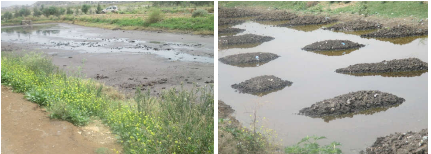
Figure 9: Sludge drying up to be converted to fertilizer in the drying bed
