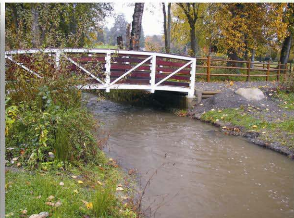
Open spaces assist in flood control
