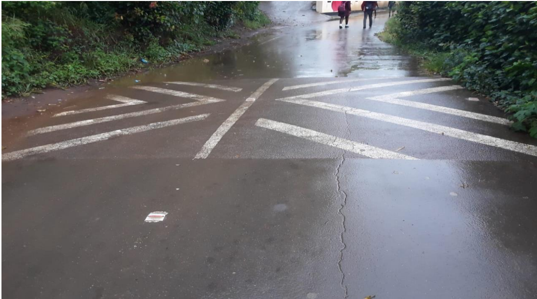
Figures 7.15: Low speed humps to slow down cars. (Source: Own).
