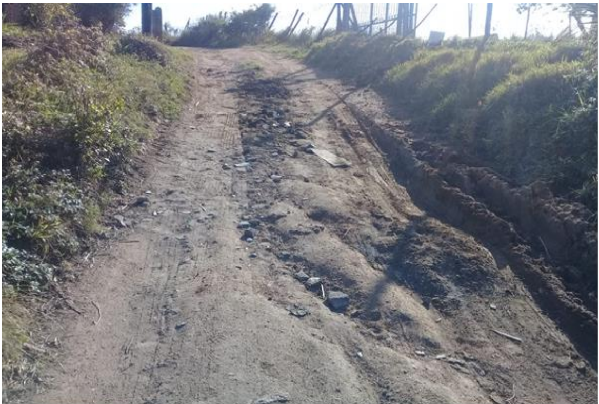
Figure 7.2: Soil erosion due to slope used as footpath by commuters. (Source: Own).
