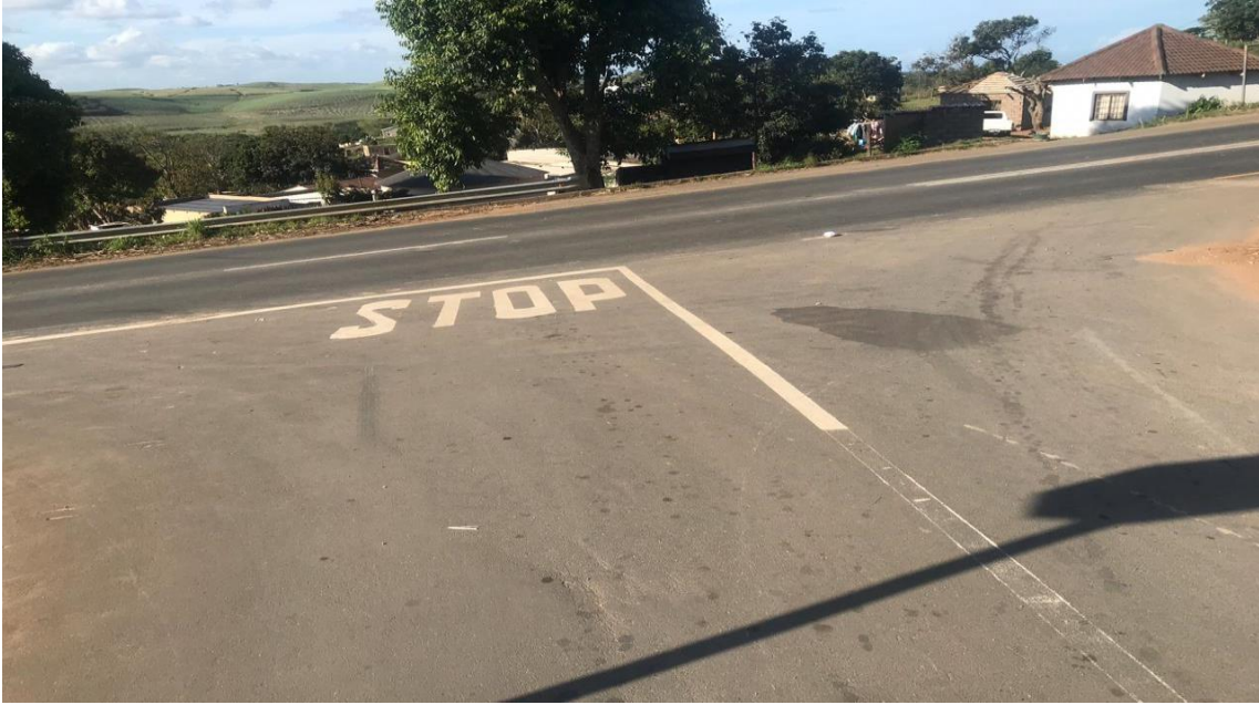
Figure 7.8: Traffic joining the provisional road here is at a disadvantage, as vehicles on the provisional road do not have to give way to them. (Source: Own).
