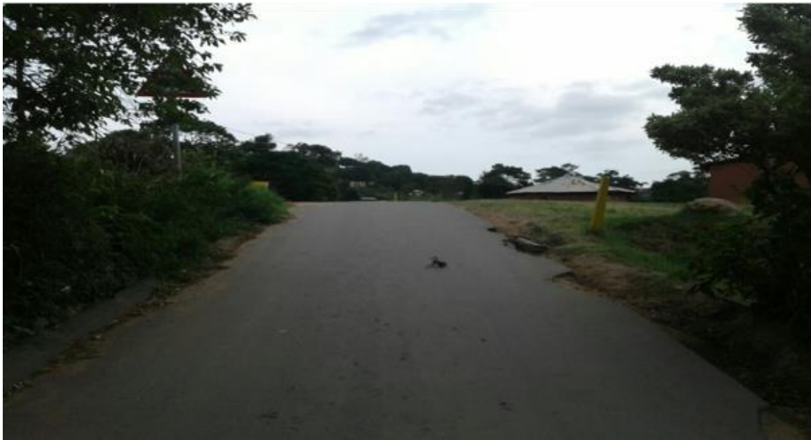
Figure 7.9: Narrow roads with blind spot corners with no safe walkways for pedestrians or enough space for two cars in opposite directions. (Source: Own).
