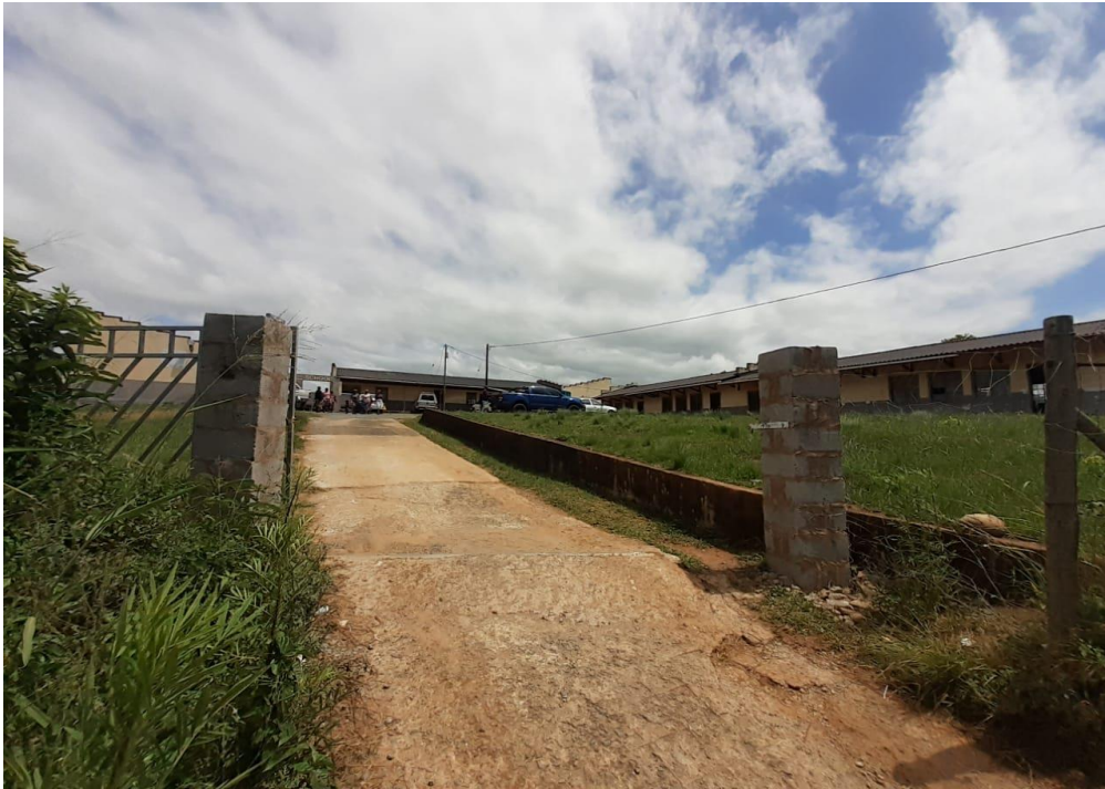
Figure 7.18: Lack of security control on who can access the school premises. (Source: Own).
