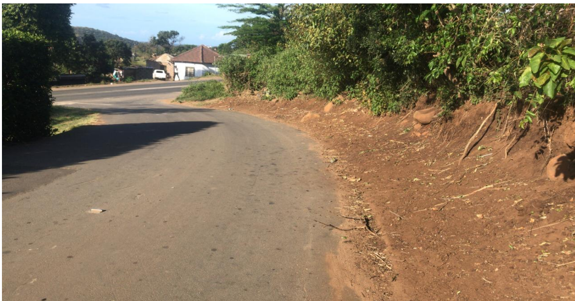
Figure 7.5: A good example of a narrow road, with a blind stop. This is a dangerous road for pedestrians to use. The ‘sidewalk’ or walkway is seldom used because it is sloped and unpaved. (Source: Own).
