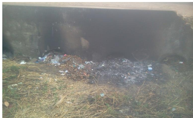
Figure 4.8: Solid waste in and around drains
