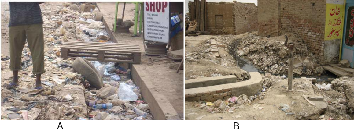
Figure 2.5: Solid waste in drains, Ota, Nigeria (A) and Rawalpindi, Pakistan (B) (Sources: Olukanni et al. , 2014; Ajaz et al. , 2010)
