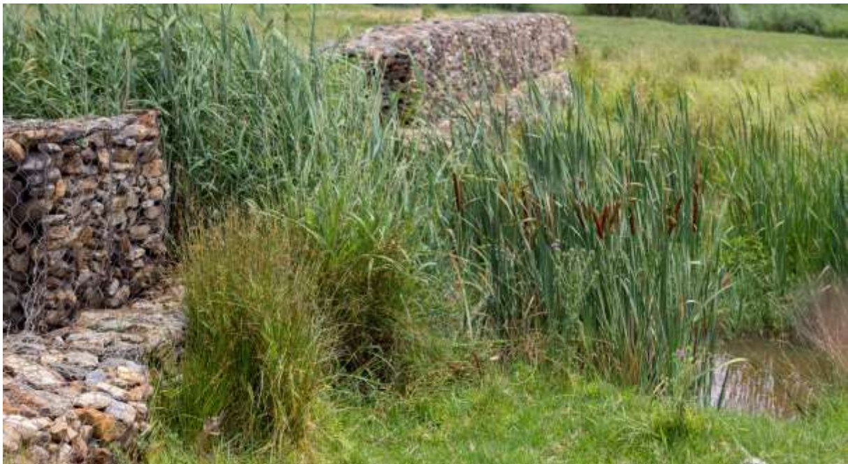
Figure 4.5: Degraded gabions erected to prevent this section of the Natalspruit from creating a second stream (especially during periods of heavy rainfall) which would undermine a road bridge (in Masakhane Street, Katlehong). Cattails are growing between the broken gabions (Source: Brits, 2018).
