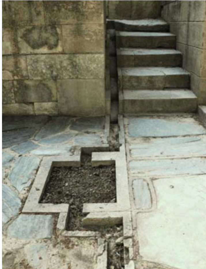
Fig. 2.24 Stepped channel for rainwater and desilting basin at Knossos (Mays 2010b:9)
