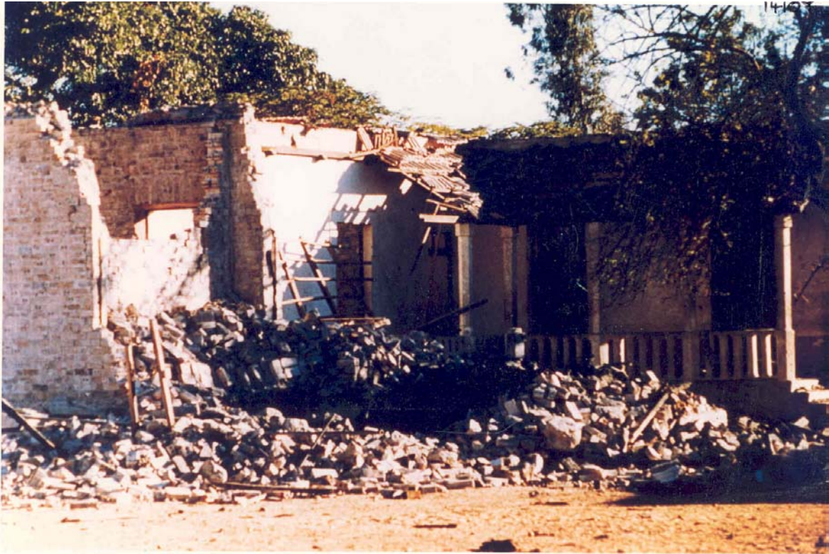
Ruins of a building destroyed at Cassinga. (Photo: Tor Sellström - National Archives of Namibia)
