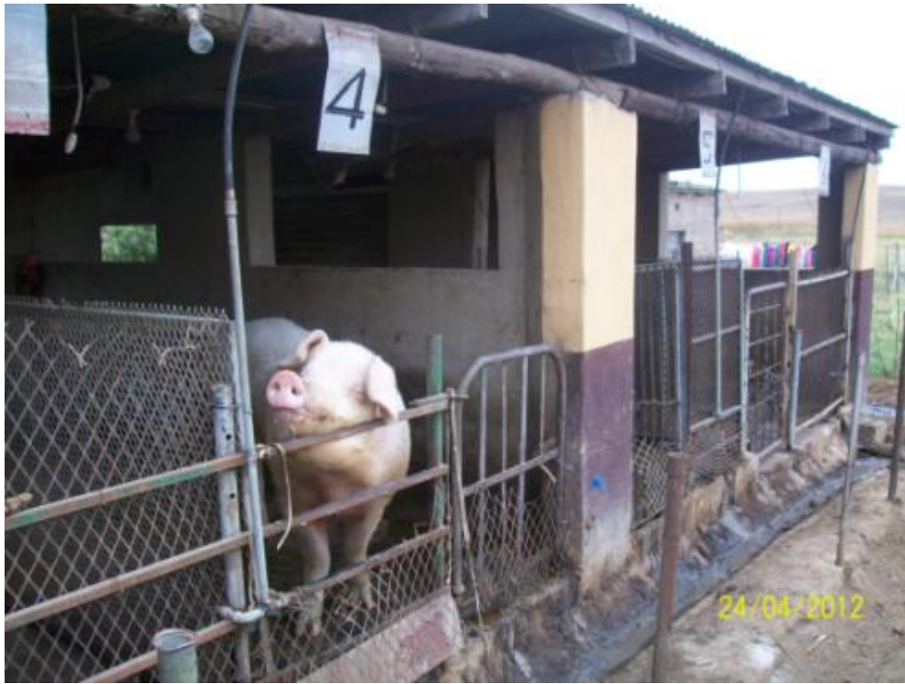
Plate 5.13: A pig house built of bricks, steel pipes and wire mesh Source: Gcumisa (2012)
