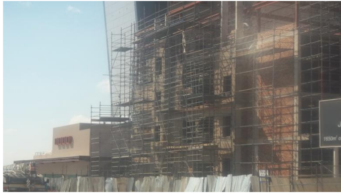
Figure 4.22a: Part of Central Business District under construction
