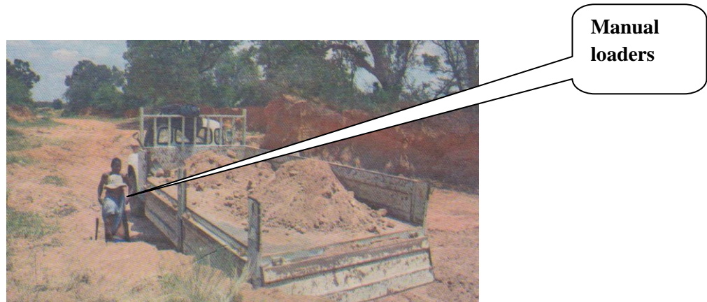
Figure 4.23: Manual loaders loading river sand into a truck using shovels
