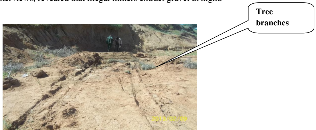
Figure 4.11: Tree branches on ground to prevent sinking on sampled Site B
