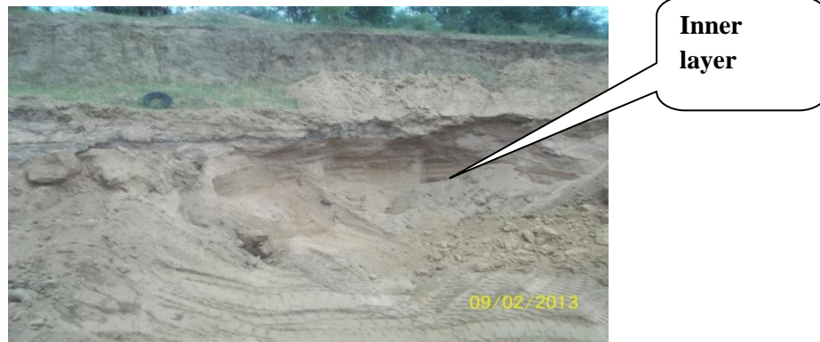
Figure 4.29: Extraction of river sand from inner layers
