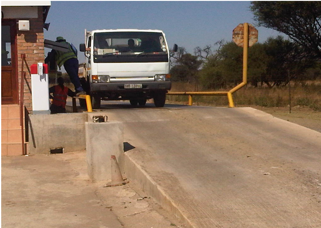
Figure 3.4: Waste weighing bridge
