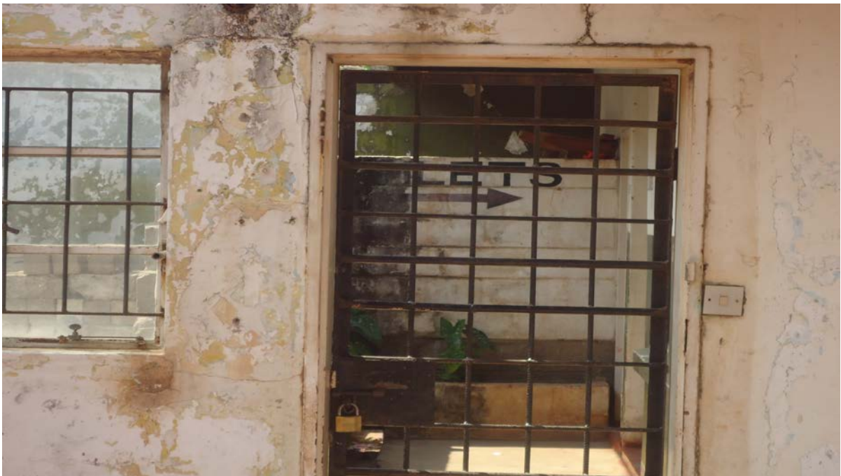
Plate 4: The toilets, outside the main building.
