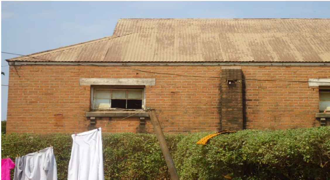
Plate 11: The outside view of the building, seen from the neighbouring premises.
