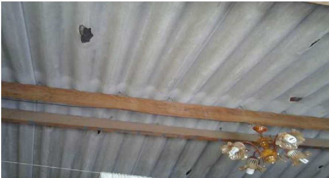
Figure 4.7 The asbestos used as a roof cover in some of the houses
