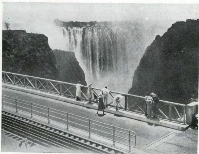
Rail and Road Bridge, Victoria Falls.
